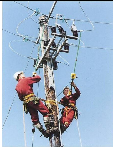
Overhead Line Testing
